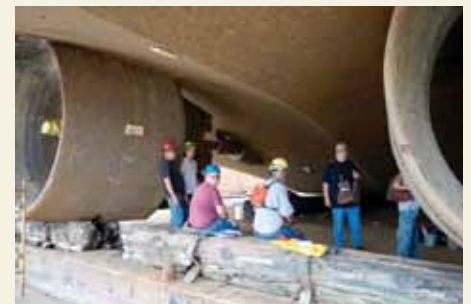
Although called "towboats" or "lineboats," these diesel-powered vessels actually push their barges. Here the artist visits the MV Sally Bromfield in a floating dry-dock where she is having two of her three rudders and one wheel (propeller) replaced. The propellers are encased in Cort Nozzles, a European invention resembling a jet's cowling designed to increase the power and efficiency of the propeller.
